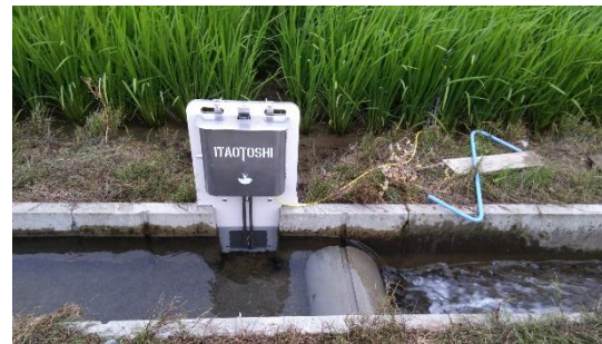
Photo 4. Raising water depth by GETAMIZU BLOCK
